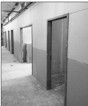
Hallway in basement level 1 once drywall is installed in late August.
